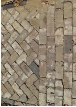
2 - Recycled brick paving
